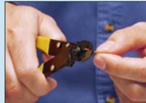
Step 1: Strip the fibre
